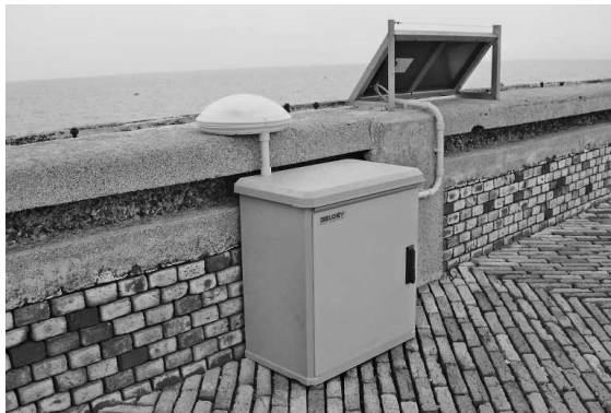
Figure 5: Fully equipped GPS measurement station on the wave breaker
